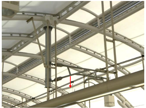
Station (ULTIMA stainless-steel clamp rod)
