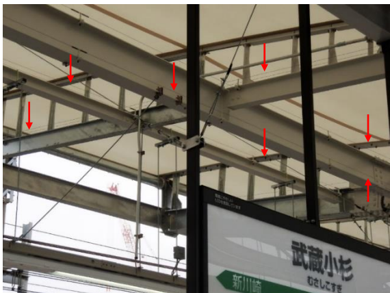
Station (ULTIMA stainless-steel clamp rod)
