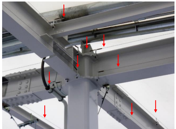
Station (ULTIMA stainless-steel clamp rod)
